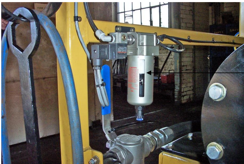
Supply Air Filter & Water Trap
